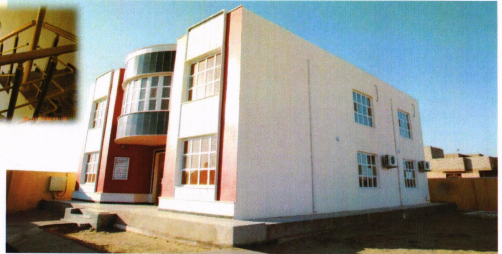
Demolition and construction of the sixth municipal section / Ramadi / Anbar
