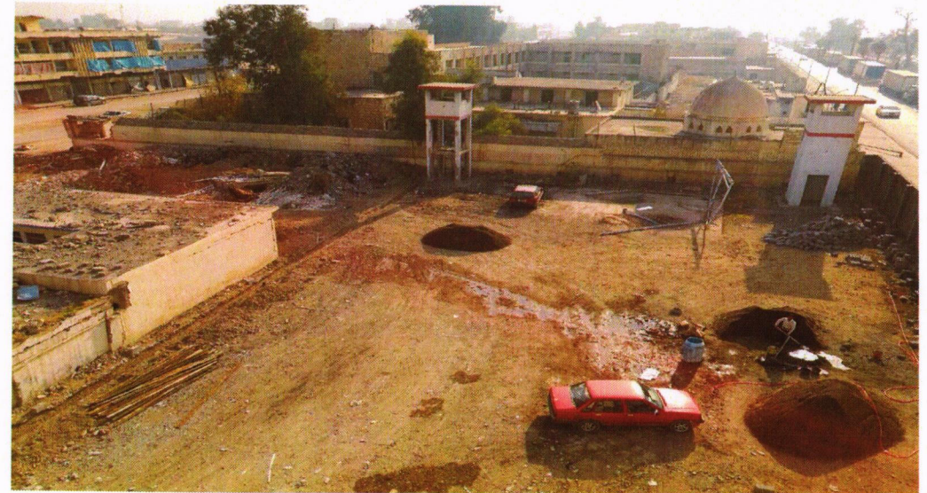
Rehabilitation of the Al nasr Police Directorate of / Nineveh
