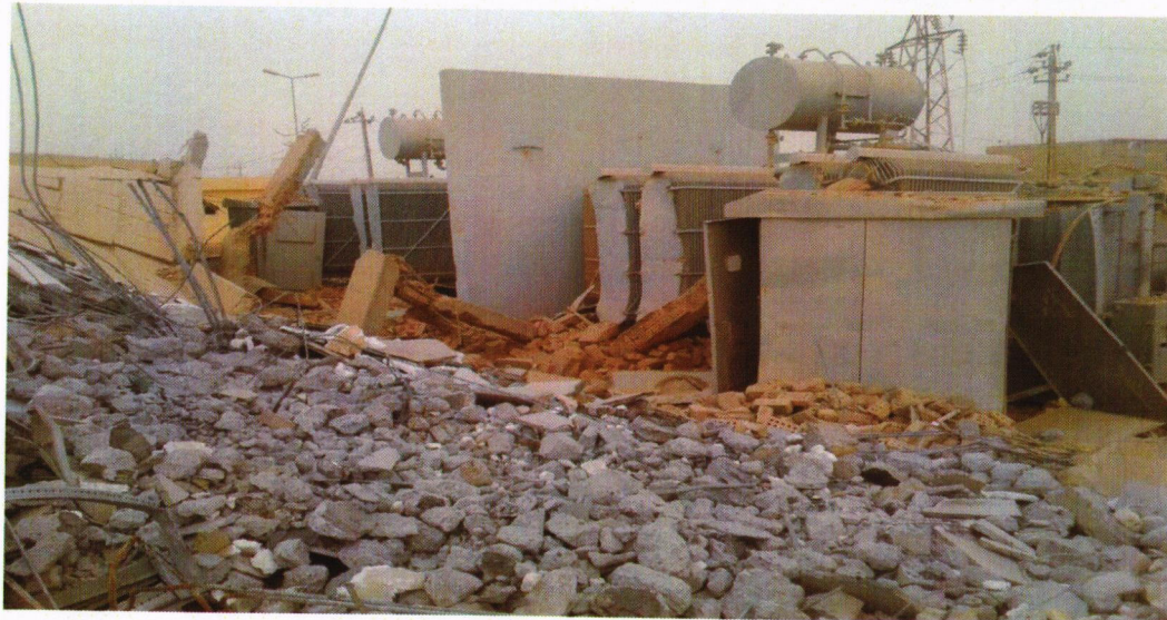
Supply and instillation Al mashtal substation 33/11 kv /heet /Al anbar
