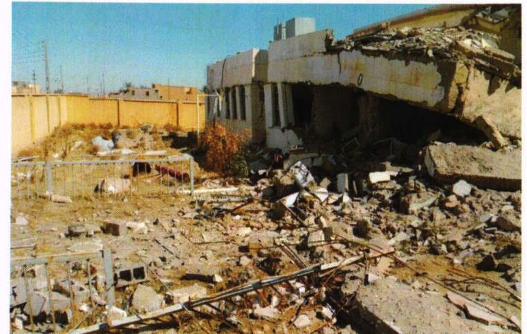
Dar AISalaam school / Heet / (before the start of construction)
