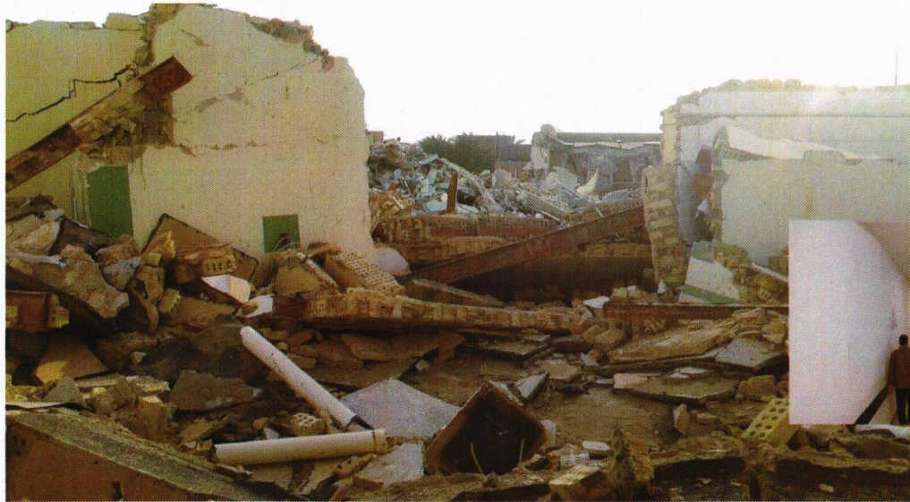
Rehabilitation of Heet General Hospital
