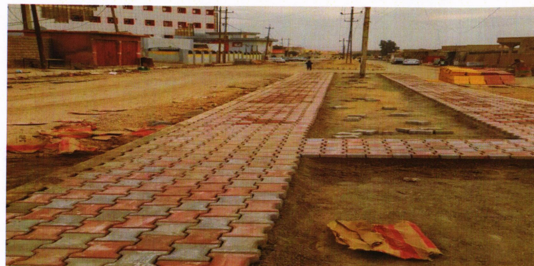
(Rehabilitation of roads (Shura area, Qayyarah, Hammam al-'Alil))
