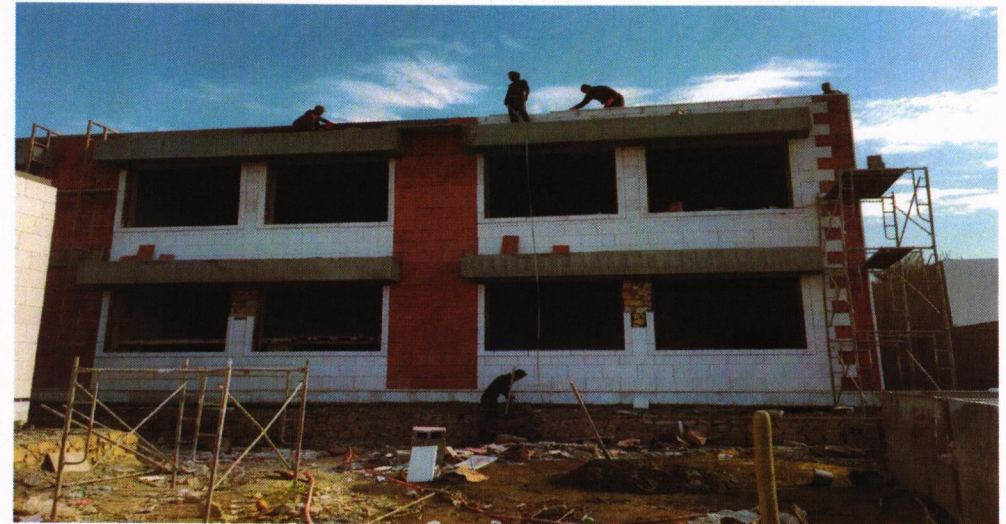
Demolition and reconstruction of al-Fatwa school / Al Anbar
