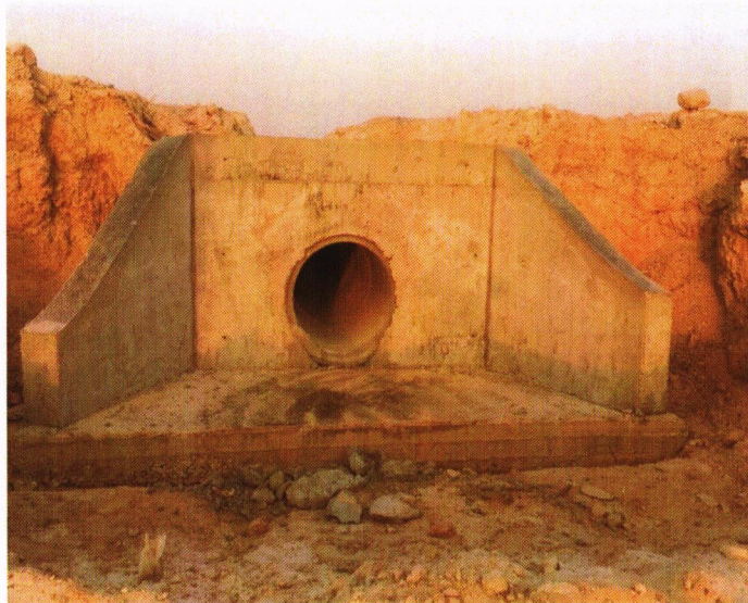
Repair and rehabilitation of a Alramadi-Heet road
