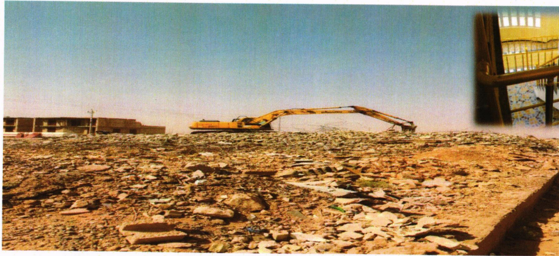
Demolition and construction of the sixth municipal section / Ramadi / Anbar
