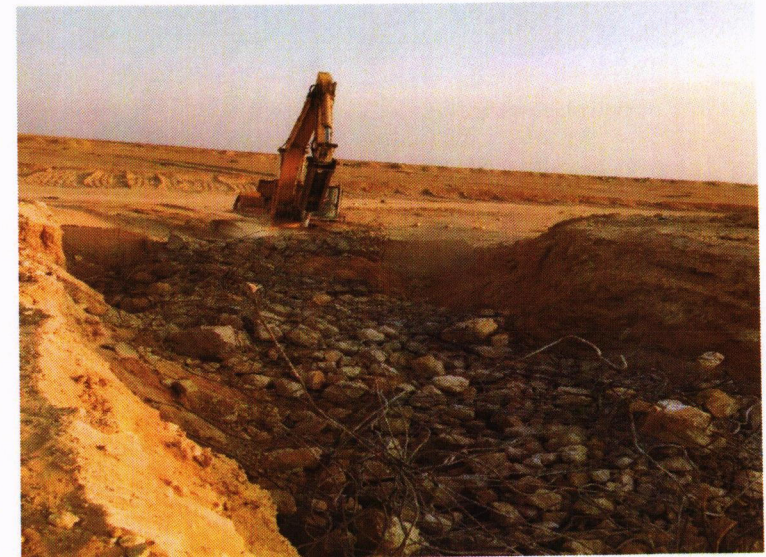
Repair and rehabilitation of a Alramadi-Hit road ( stage of work)
