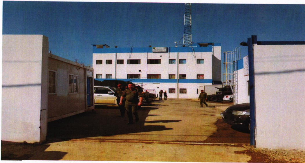
Rehabilitation of the Al nasr Police Directorate of / Nineveh
