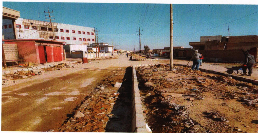
(Rehabilitation of roads (Shura area, Qayyarah, Hammam al-'Alil))
