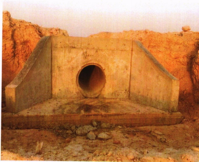
Repair and rehabilitation of a Alramadi-Heet road
