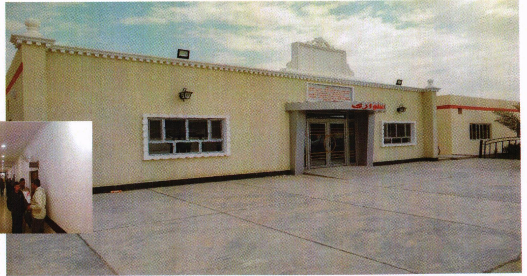
Rehabilitation of Heet General Hospital
