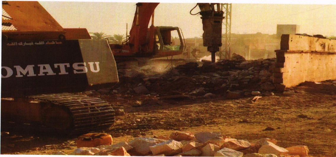
Demolition and reconstruction of al-Fatwa school / Al Anbar
