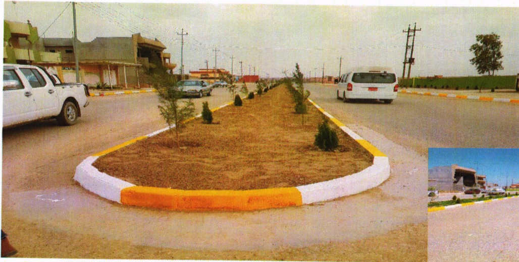
Rehabilitation of roads in Hamdania and Nimrod / Nineveh
