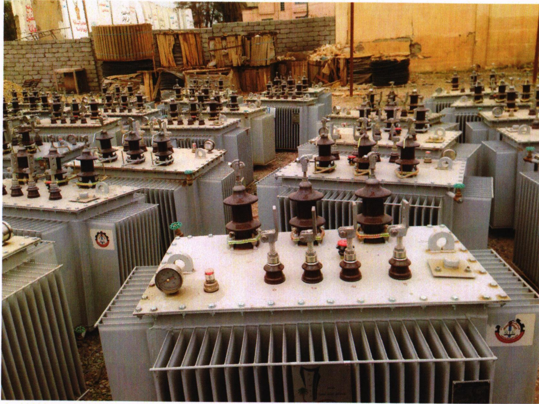
supply of power transformers to the right side/mosel
