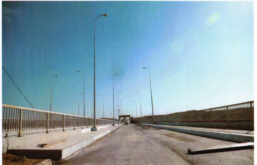
Rehabilitation of the Shishin Bridge\ Salah Al Din
