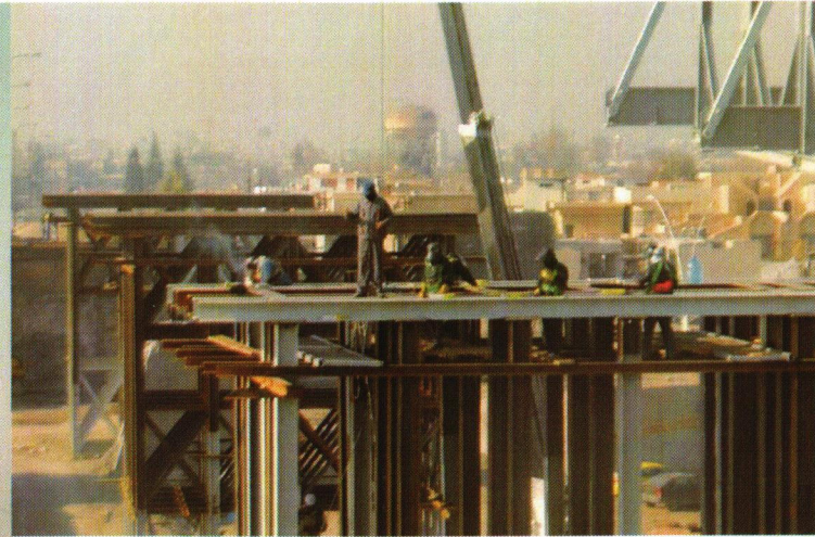
Temporary solution for Mosul Forth Bridge
