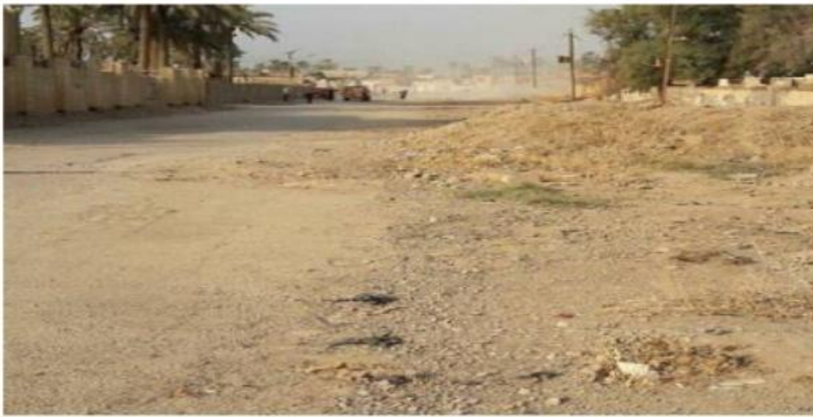
Rehabilitation and Building Al Souq Street /Saadia/Diyala (before starting)
