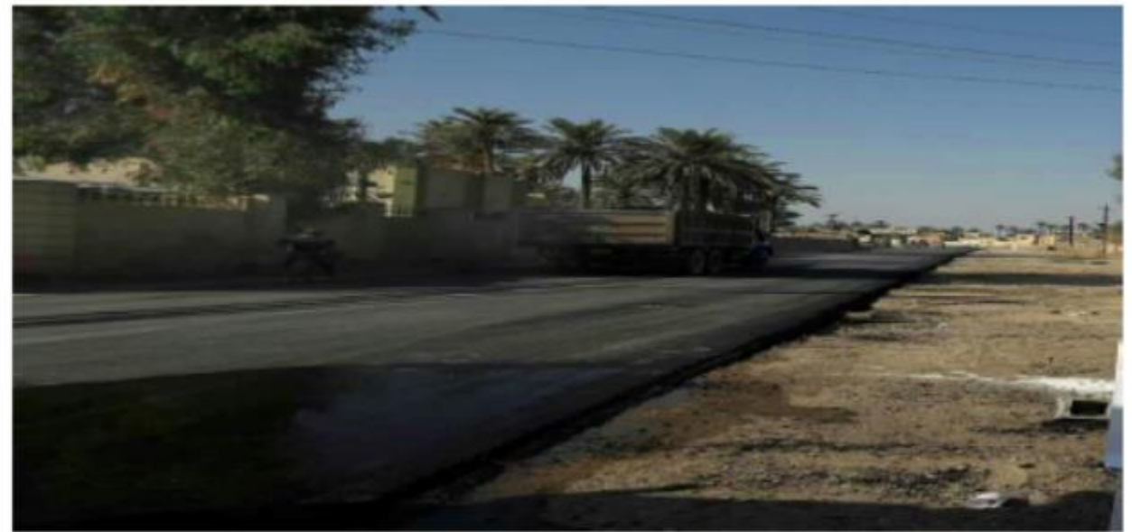
Rehabilitation and Building Al Souq Street /Saadia/Diyala (completion of work)
