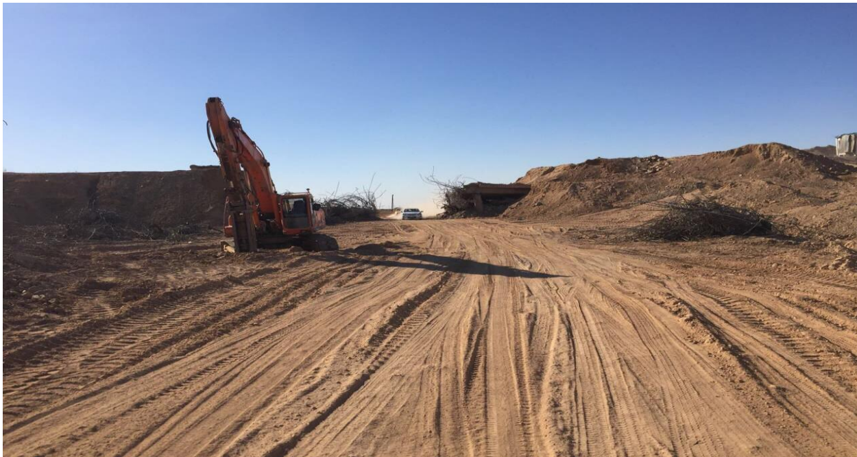
Rehabilitation and paving of Kirkuk - Hawija road near Mujaser Khalid
