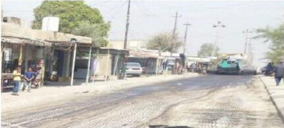
Building of the Road (Al Hamia – Snedeej) / Jurf Al Nasr/Babil (before starting)
