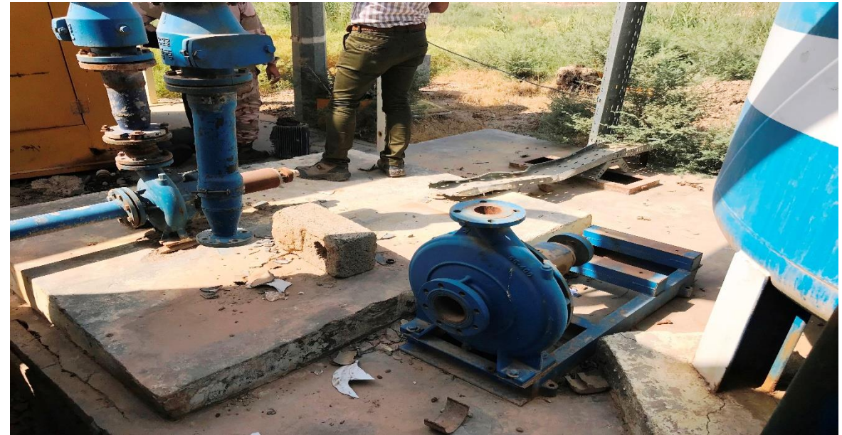
(Rehabilitation of Al Hitaween water station/Abu ghraib/ Baghdad belt)
