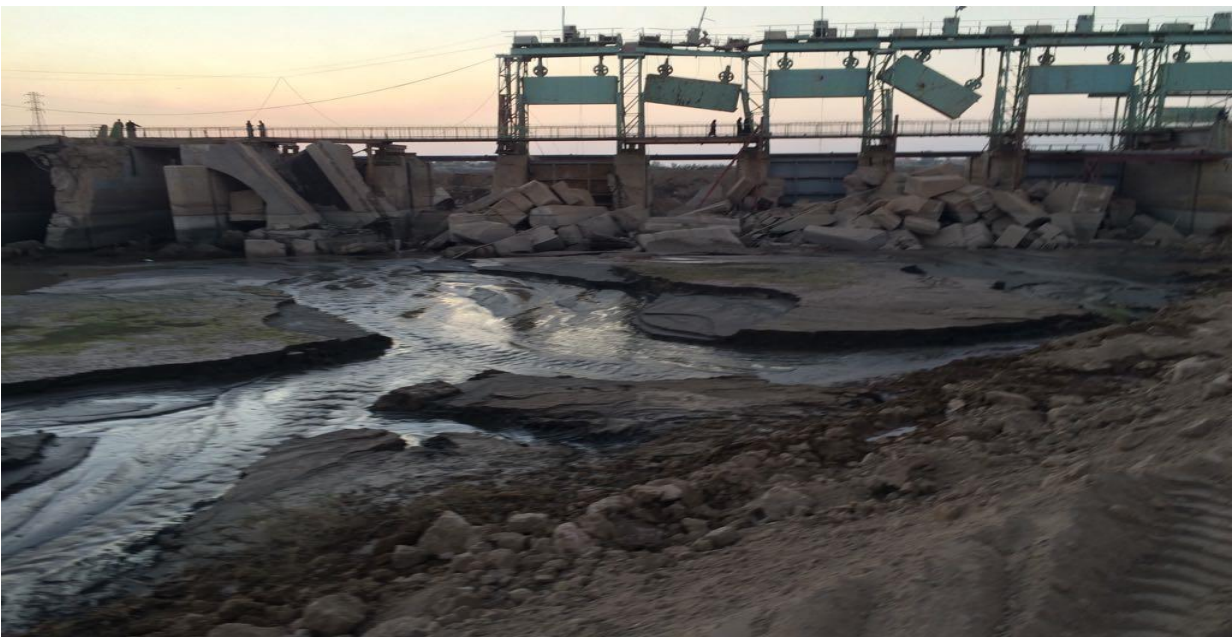
Reconstruction of Ramadi dam on the Euphrates River / Ramadi / Anbar
