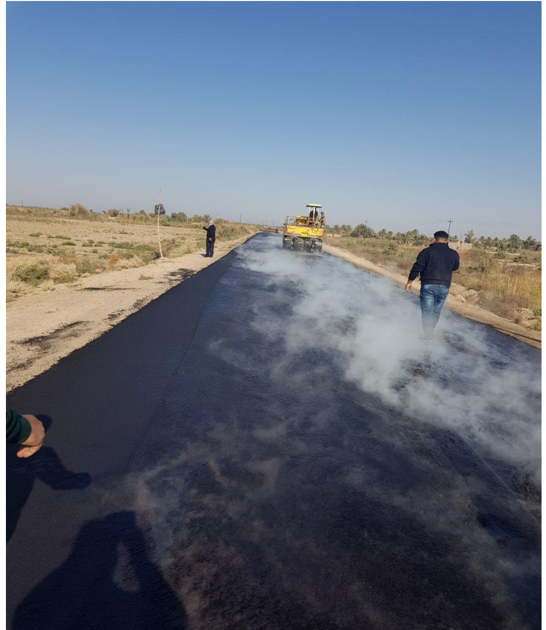
Al Khidar road along the Euphrates River for 18 km
