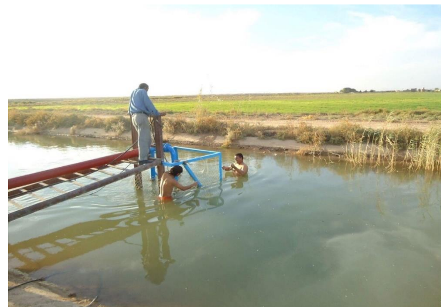
Rehabilitation of Mezher Al - Asi water station / Hawijah
