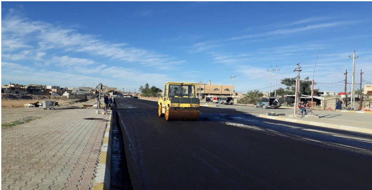
Rehabilitation of the main public street / Jalawla / Diyala
