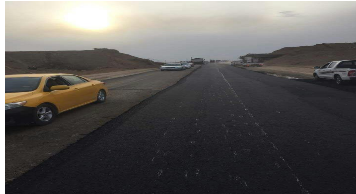
Rehabilitation and paving of Kirkuk - Hawija road near Mujaser Khalid
