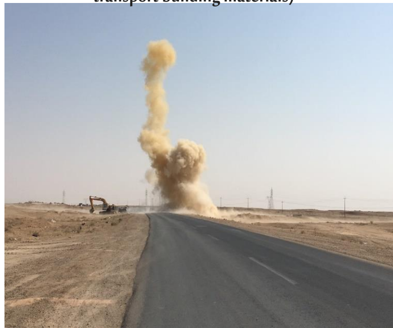
Repair and rehabilitation of a Alramadi-Heet road ( a bomb explosion)
