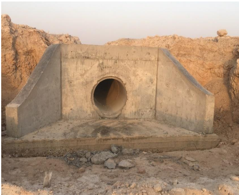
Repair and rehabilitation of a Alramadi-Heet road
