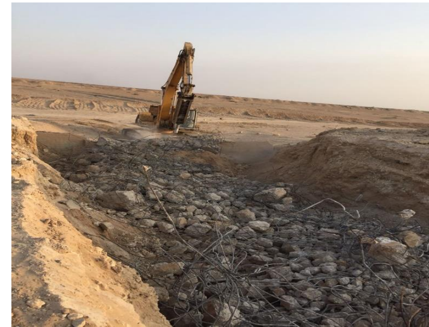
Repair and rehabilitation of a Alramadi-Hit road ( stage of work)
