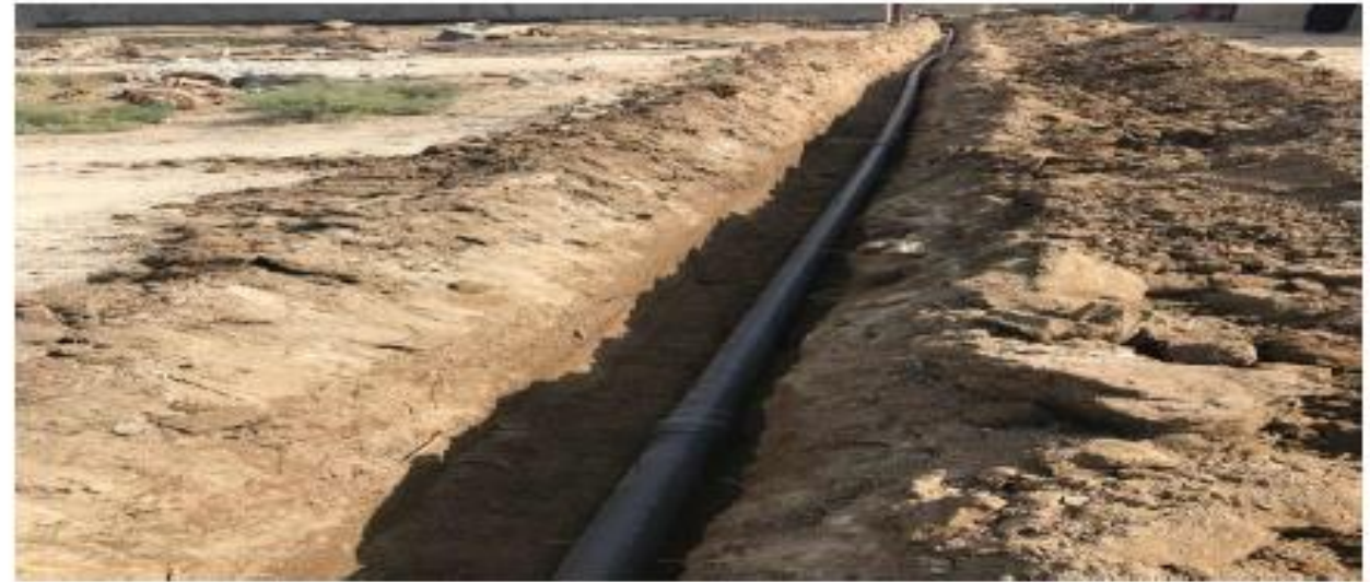
Replacement of the water network / North Babylon (stage of work)
