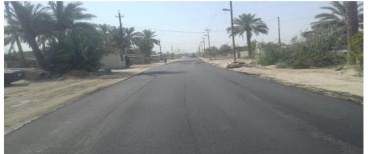
Building of the Road (Al Hamia – Snedeej) / Jurf Al Nasr/Babil (Completion of work)
