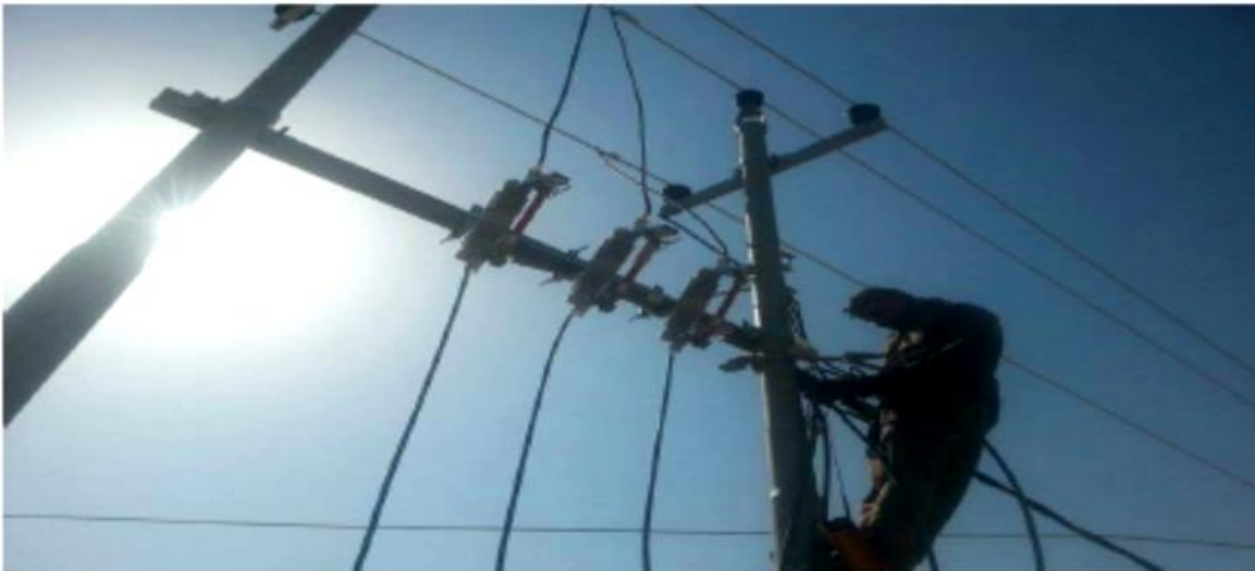
Rehabilitation of Electrical networks in the village of Mullah Abdullah/ Kirkuk
