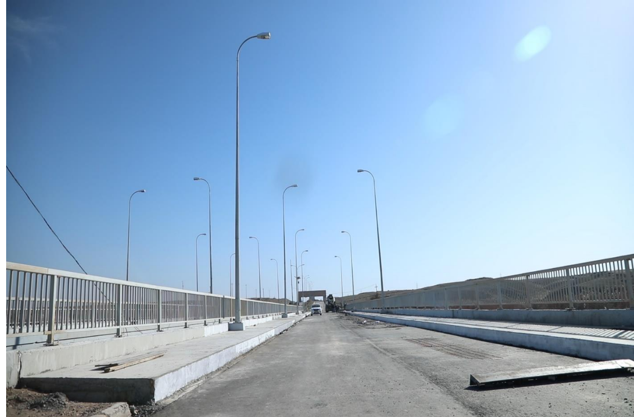
Rehabilitation of the Shishin Bridge\ Salah Al Din
