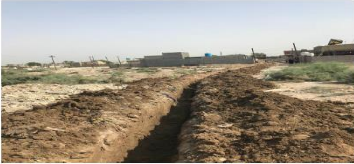
Replacement of the water network / North Babylon (stage of work)
