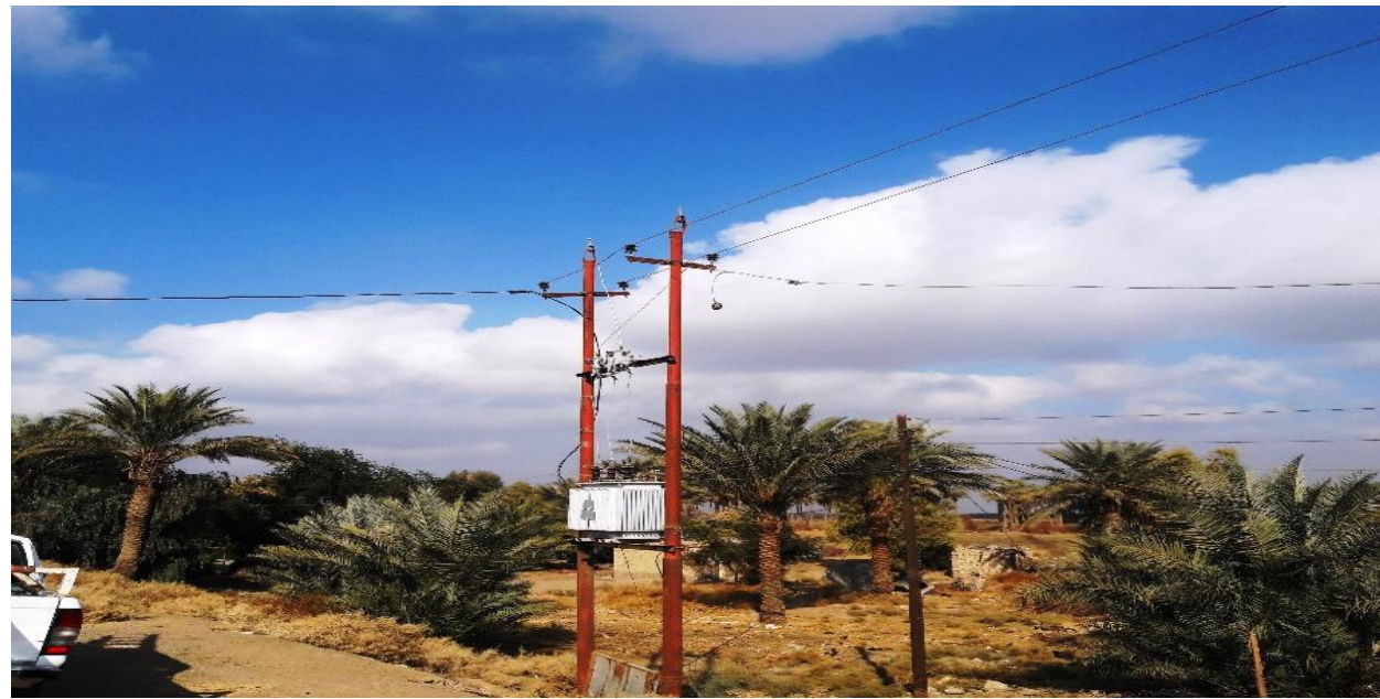
Rehabilitation of electrical network in abu ghraib villages / Baghdad belt
