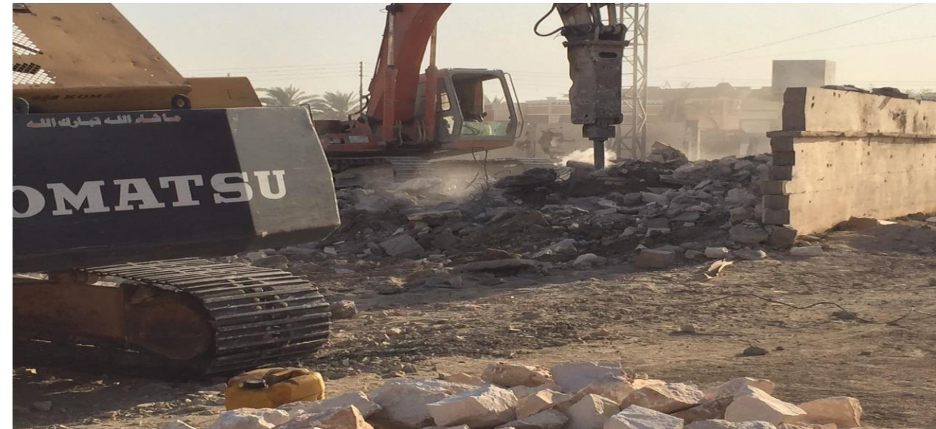
Demolition and reconstruction of al-Fatwa school / Al Anbar
