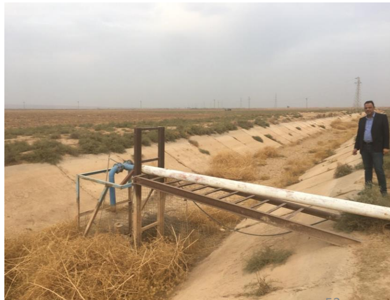
Rehabilitation of Mezher Al - Asi water station / Hawijah
