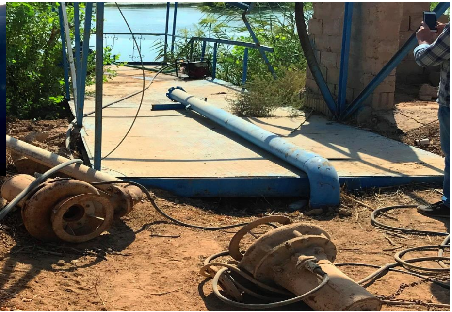
(Rehabilitation of Al Sadaan water station/Abu ghraib/ Baghdad belt)
