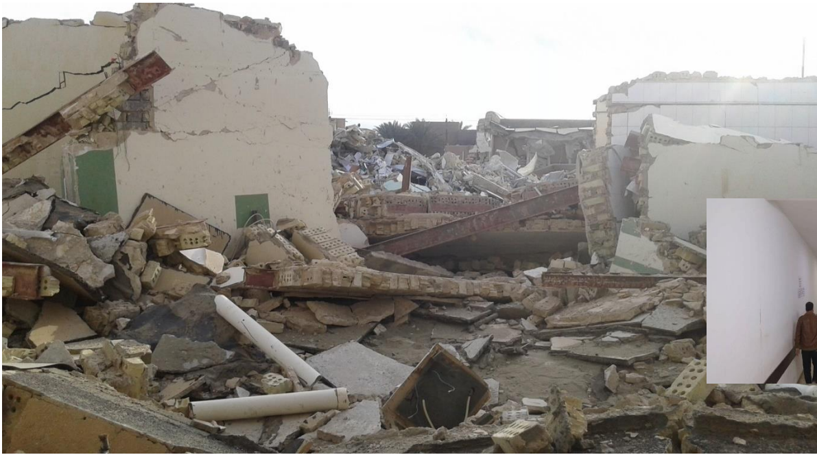
Rehabilitation of Heet General Hospital
