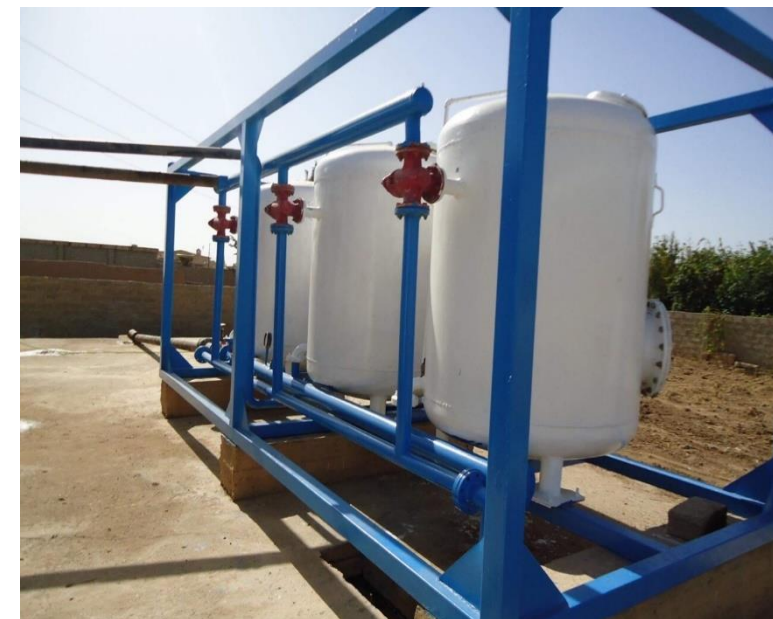
Rehabilitation of Mezher Al - Asi water station / Hawijah
