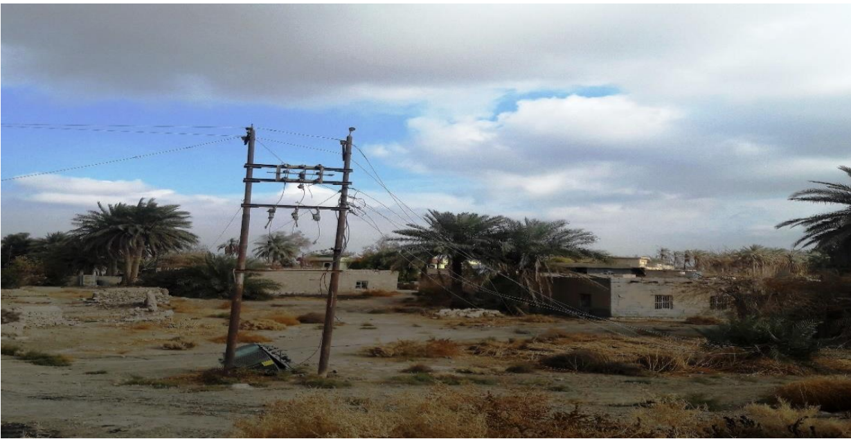
Rehabilitation of electrical network in abu ghraib villages / Baghdad belt
