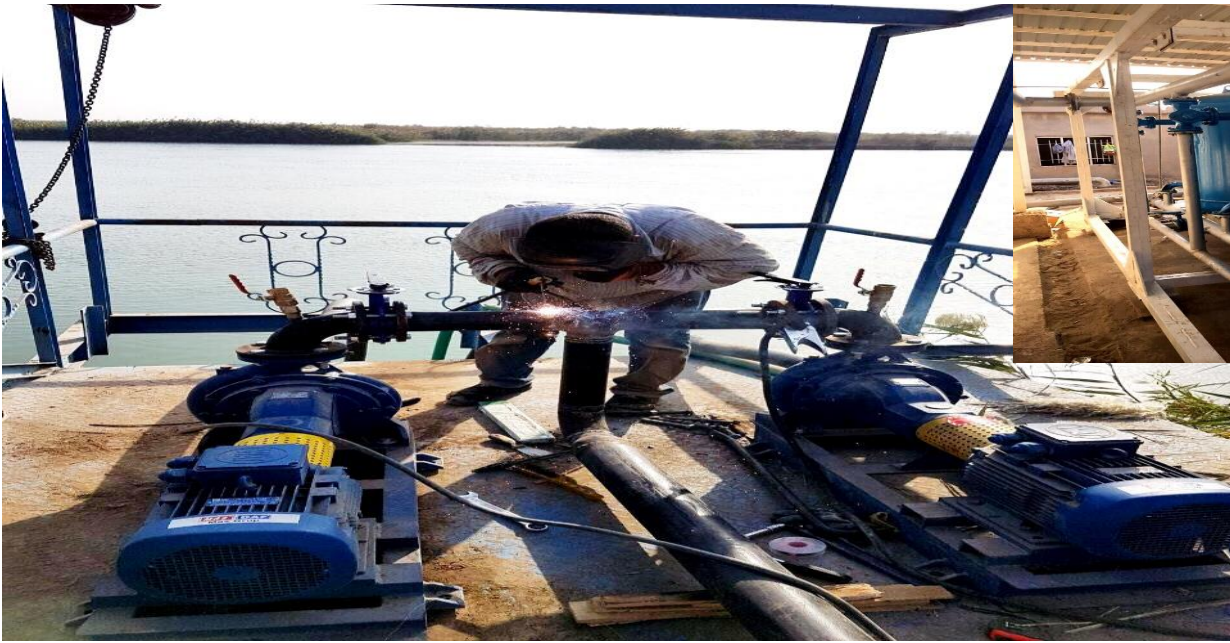
(Rehabilitation of Al Sadaan water station/Abu ghraib/ Baghdad belt)
