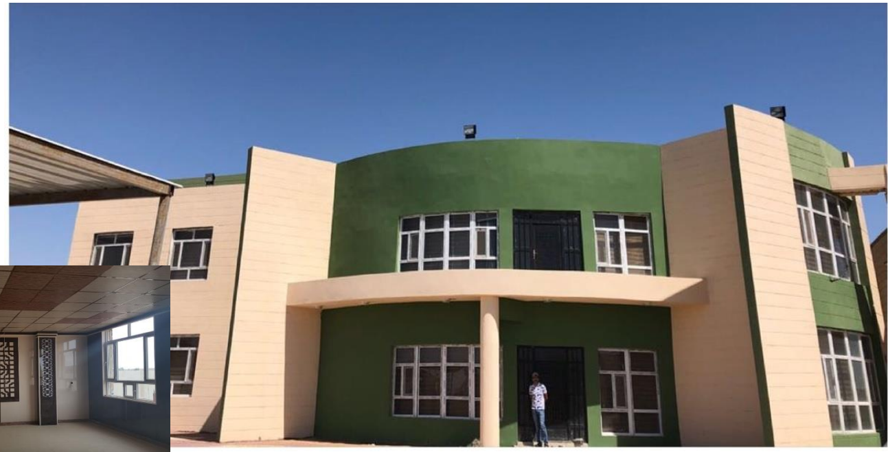
Rehabilitation of the dejlah district building /samarra/salah al din
