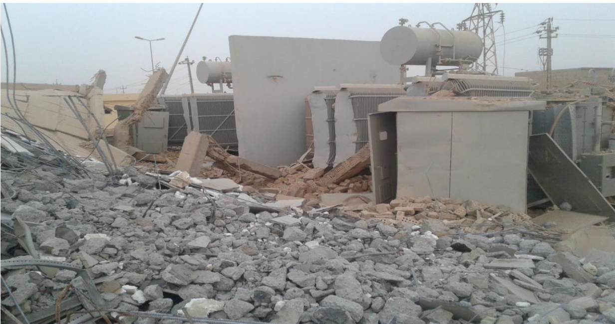
Supply and installation Al mashtal substation 33/11 kv /heet /Al anbar
