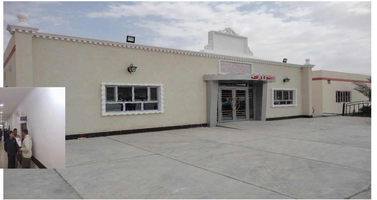
Rehabilitation of Heet General Hospital
