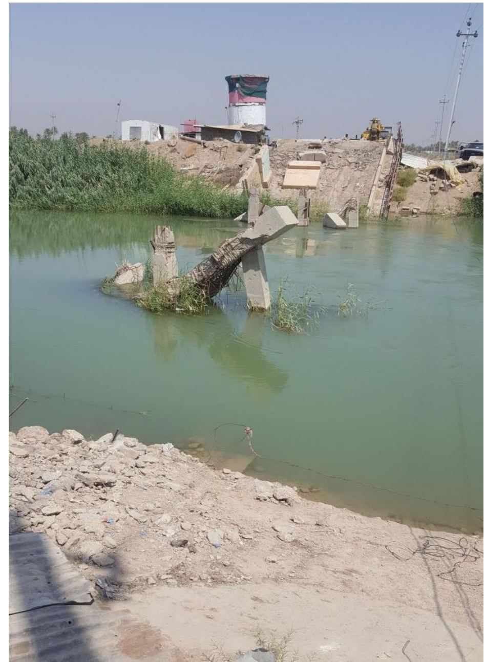
Awdat Al Shukr bridge/abu ghraib/Baghdad belt
