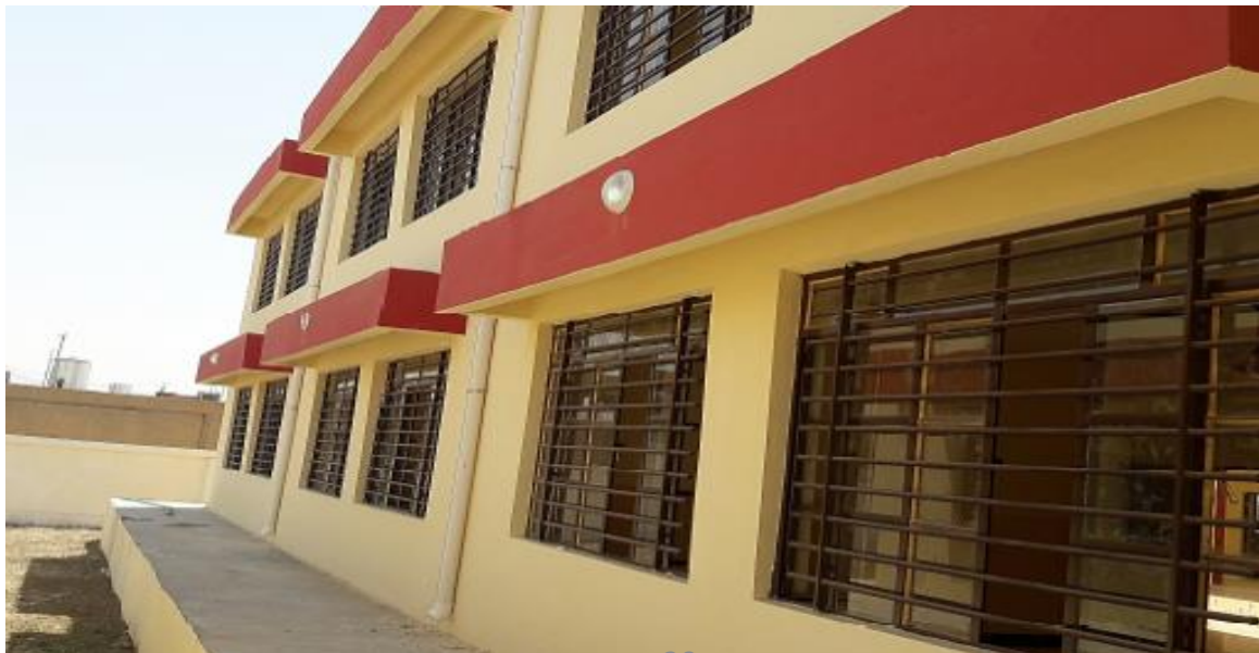
Al-Qayyarah Preparatory School / Al Qayyarah / Nineveh
