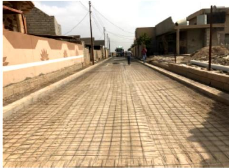
Rehabilitation and Building of streets in Al Bashir village / Kirkuk (stage of work)
