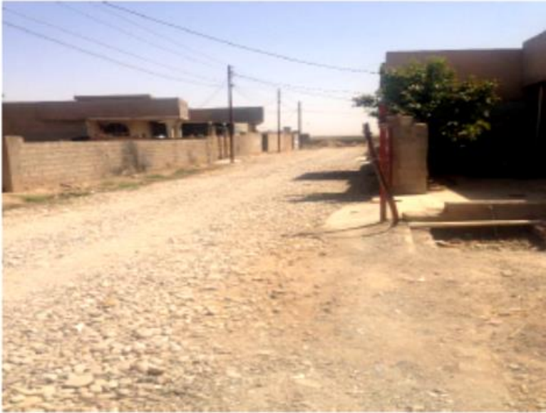
Rehabilitation and Building of streets in Al Bashir village / Kirkuk (Before starting)
