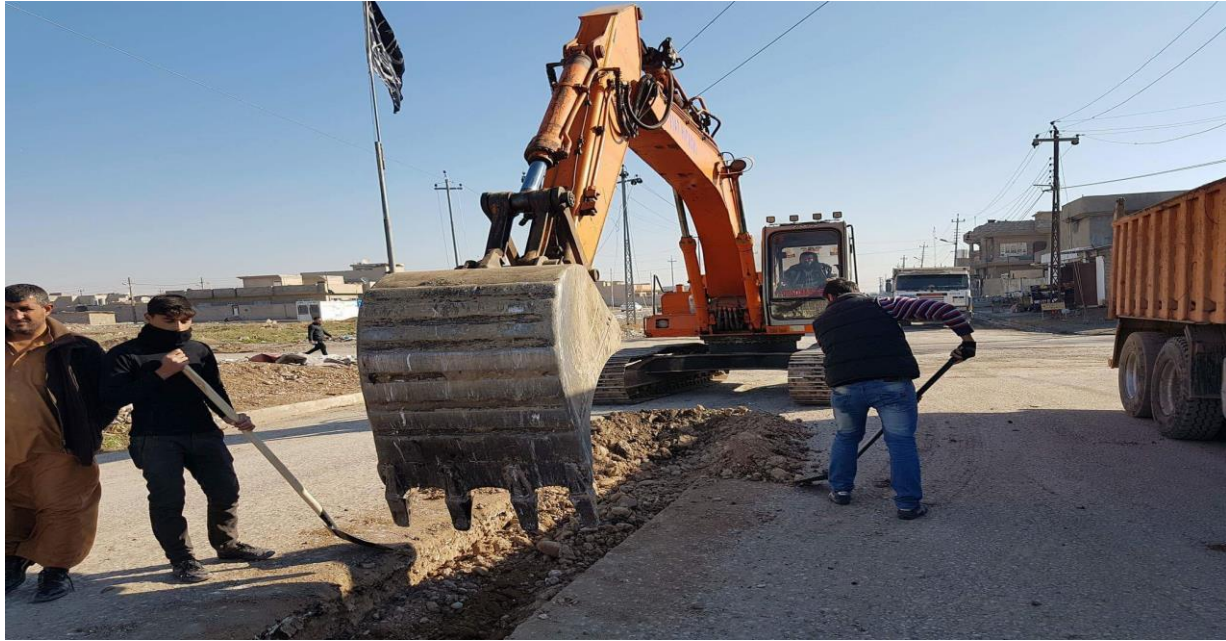
(Sewage system and pavement works / Bartala and Baishika)
