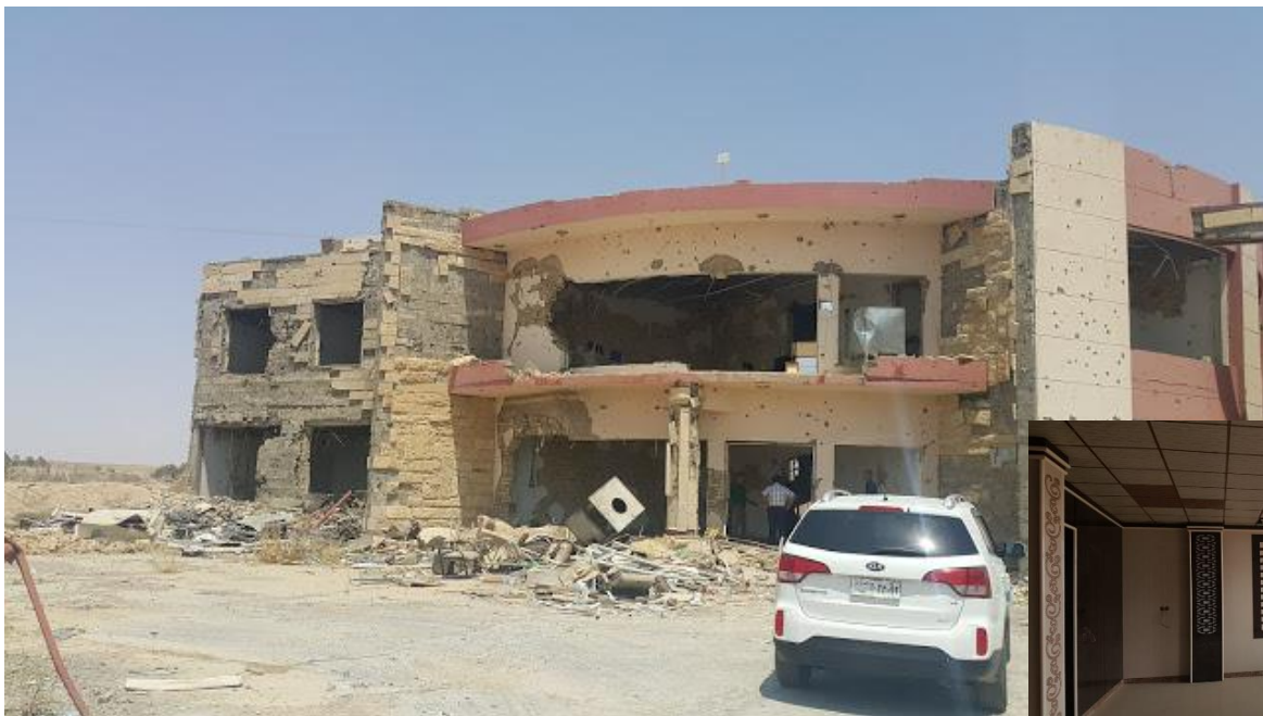
Rehabilitation of the dejlah district building /samarra/salah al din
