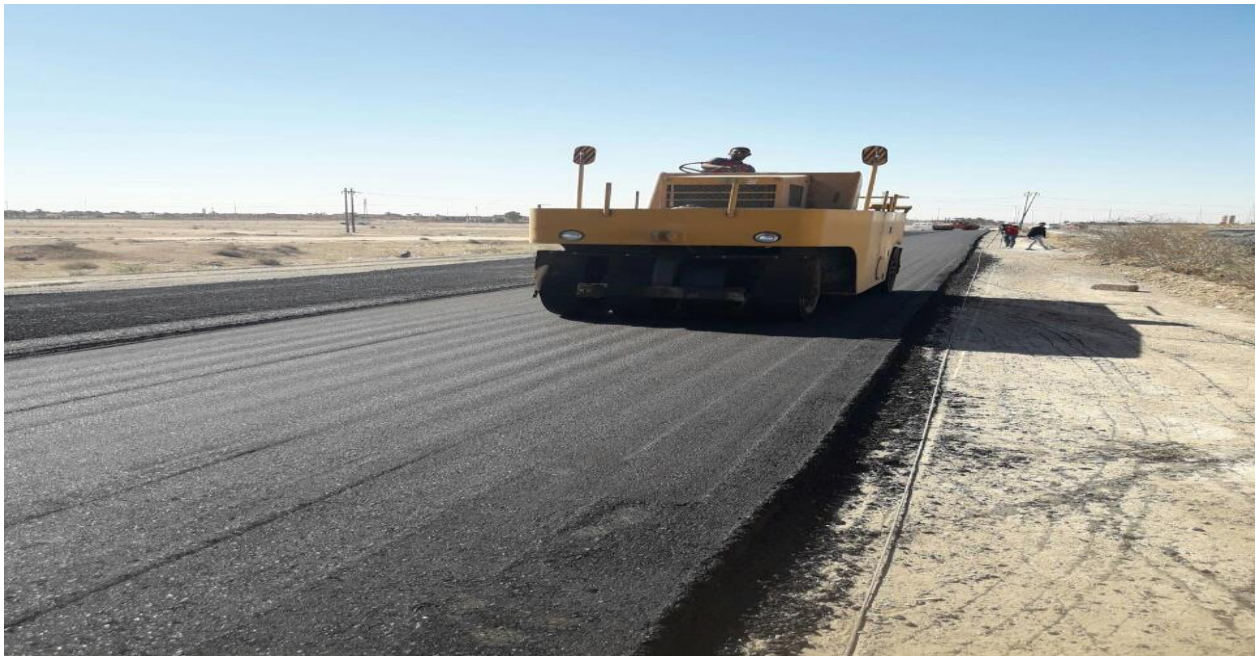
Rehabilitation of Al Dur institute street /Salah Aldin
